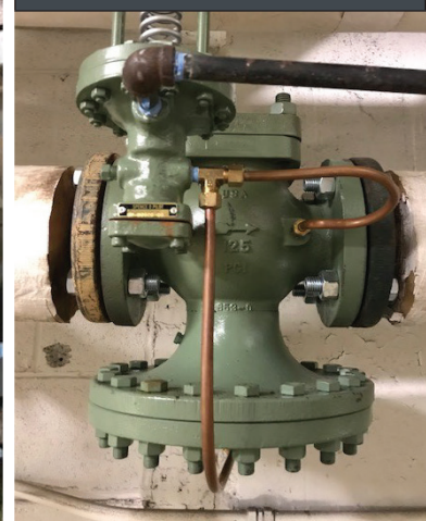
NEW STEAM PRESSURE-REDUCING VALVE STATION
