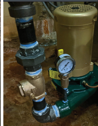
NEW STEAM PRESSURE-REDUCING VALVE STATION
